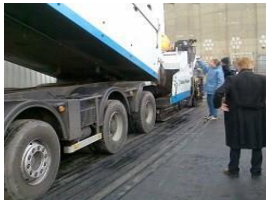
Hot laying with asphalt machine
