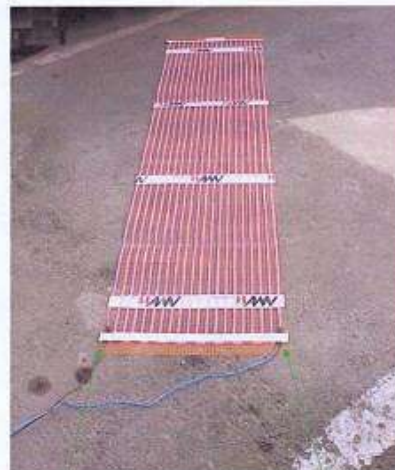
Input Voltage connection point.
